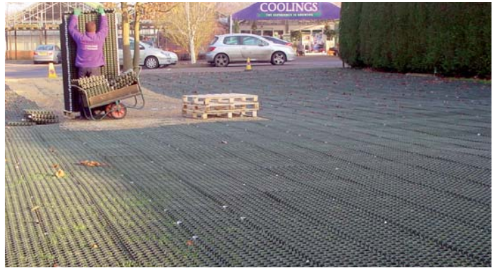
BodPave® installation for a grassed overflow car park
