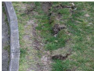
Roadside rutting & damage
