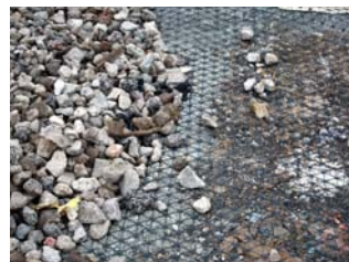
Geogrid layer installed
